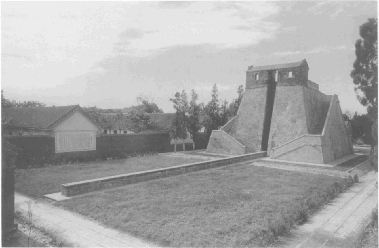
FIG. 3.21. YUAN OBSERVATIONAL TOWER. This observational tower in Dengfeng Xian (in present-day Henan Province) once contained a gnomon about twelve meters tall. Extending horizontally on the ground from the north side of the tower is a graduated scale more than thirty-six meters long, which was used to measure the sun's shadow.
