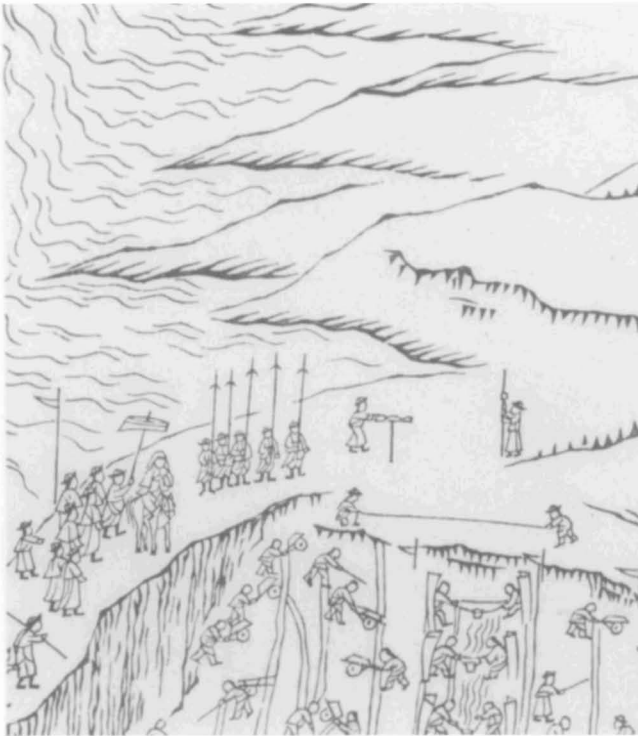
FIG. 5.4. WATER CONSERVANCY WORKERS PERFORMING MEASUREMENTS FOR CUTTING A CANAL. This is a detail from a Qing illustration.
